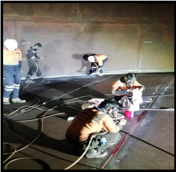
Visual inspection & DPT
