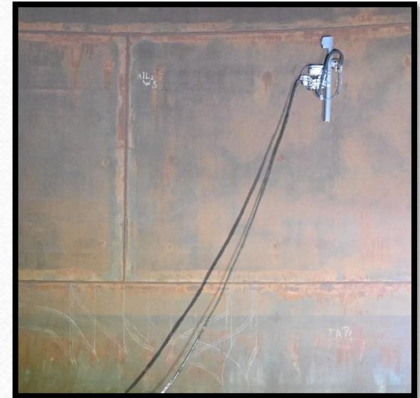
Corrosion mapping test
